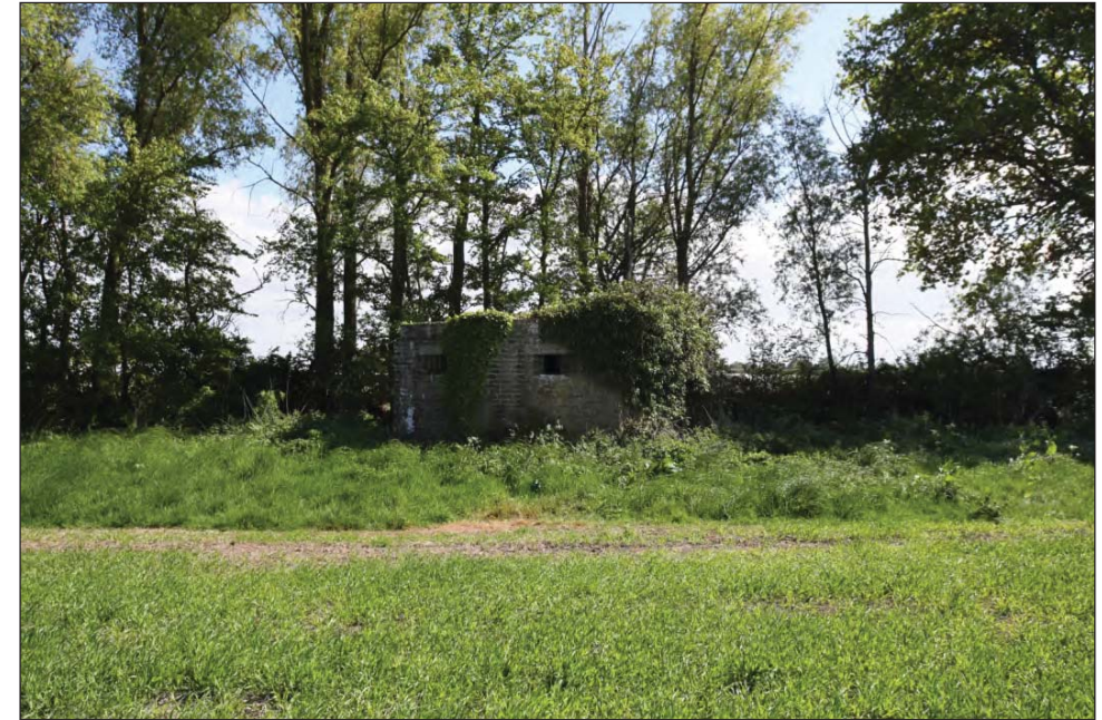
Plate 59: View of Pillbox at the southern edge of Parcel 16 (WA75)
