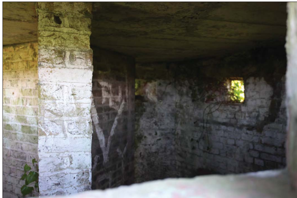
Plate 62: View looking through gun emplacement at internal anti-ricochet wall
